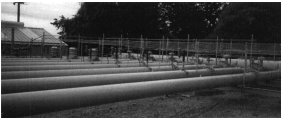
Figure 5-6 Good design calls for long, straight meter tube lengths for the most accurate flow measurement with minimum uncertainty.
