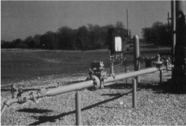
Figure 13-2 Typical orifice meter installation.
