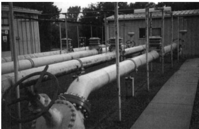
Figure 3-2 Typical meter and regulation station components.
