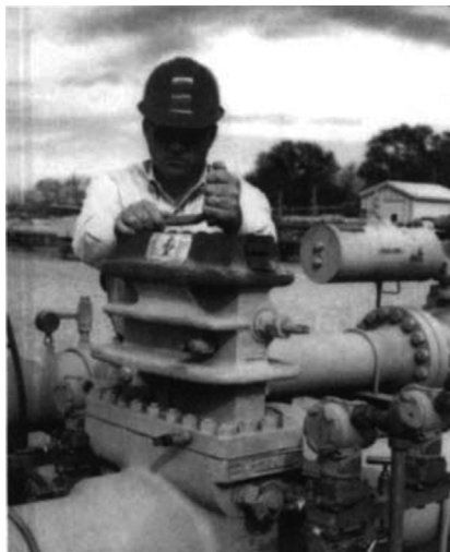
Figure 5-11 Meters and meter tubes must be properly maintained for accurate flow measurement.
