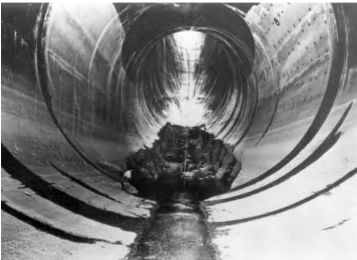
Figure 6.5. Cavitation damage to the concrete wall of the 15.2 m diameter Arizona spillway at the Hoover Dam. The hole is 35 m long, 9 m wide, and 13.7 m deep. Reproduced from Warnock (1945).
