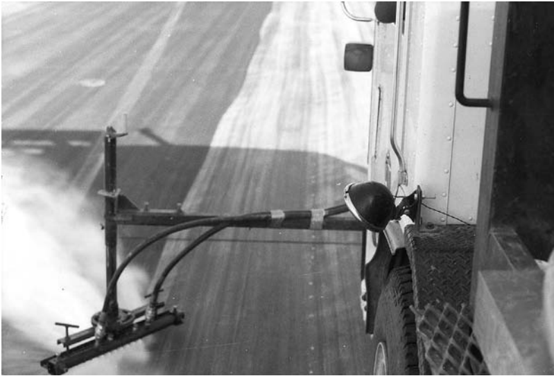
Figure 12.15. Rubber removal in Saudi Arabia ( G. Pegoda )
