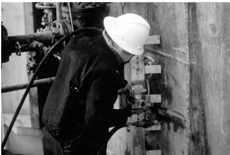
Figure 7.4. Cutting steel and refractory on reactor vessel ( Courtesy of HydroChem )
