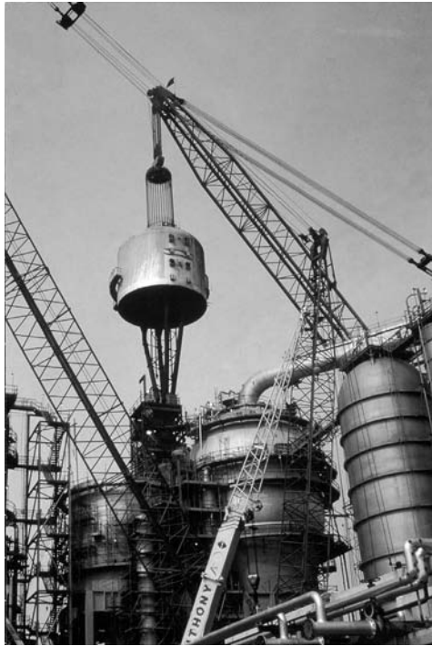
Figure 7.5. Lifting the top of a reactor vessel ( Courtesy of HydroChem )
