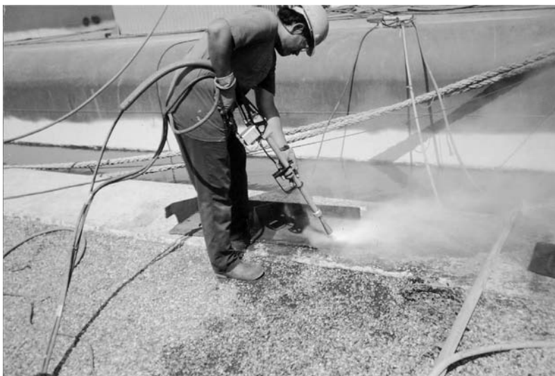
Figure 8.2. Operator testing ultra-high pressure handgun for coating removal
