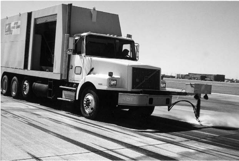
Figure 12.10. Runway cleaning operation (Courtesy of Aqua-Dyne)
