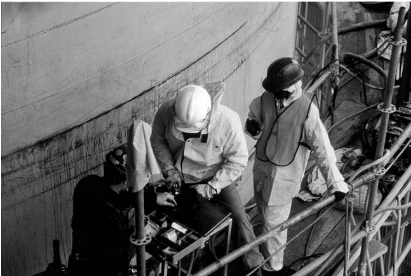
Figure 7.3. Installing cutting equipment on reactor vessel ( Courtesy of HydroChem )
