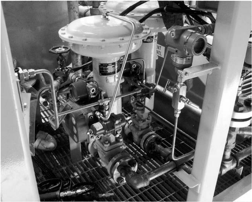
Figure 10.3. Air-operated high temperature relief valve
