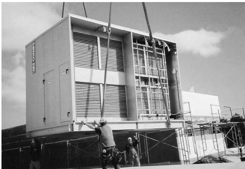
Figure 7.28 A heat pipe heat exchanger with spray bars (visible on the RHS). These are used on the exhaust side for indirect evaporative cooling, in addition to sensible heat transfer.
