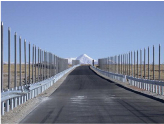
Figure 7.34 The Tibet–Qinghai highway, showing thermosyphons to preserve the embankment on each side of the road. They are protected by crash barriers [70].
