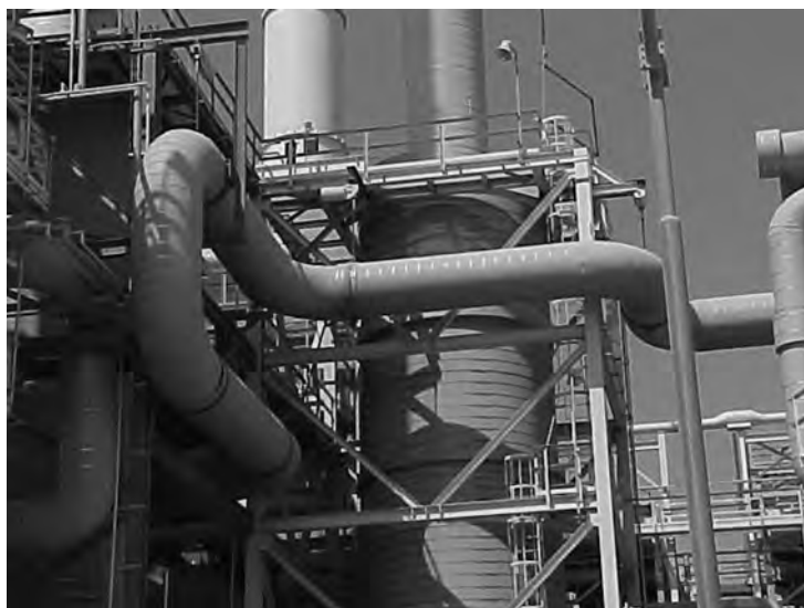
Figure 5-8a. A typical piping supported by constant spring hangers. The 36" \phi header is an ethyl benzene line that operates at 893°C (1639.4°F). The line has large thermal growth and "floats" with the constant springs. Adjusting the springs was like the "waterbed" phenomenon, which is described later. These springs were known as "the seven sisters." The pipe material is Incoloy.
