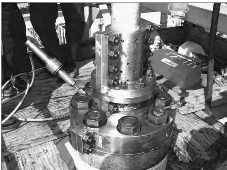
Figure 6-30c. Photo of clamp installed and injecting sealant.
