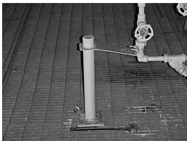
Figure 5-15. Flexible beam support in operating hot condition.
