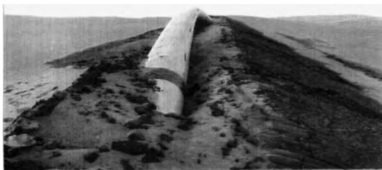
Figure 8-23a. Top view of bowing of a trunkline in the desert.
