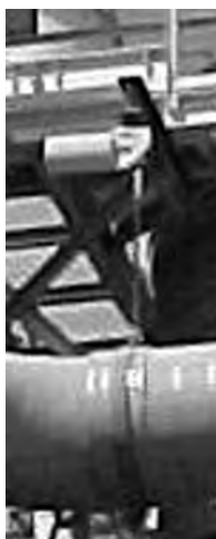
Figure 5-8b. Insert of one of the seven constant spring hangers of the 36" \phi header shown in Figure 5-8a .
