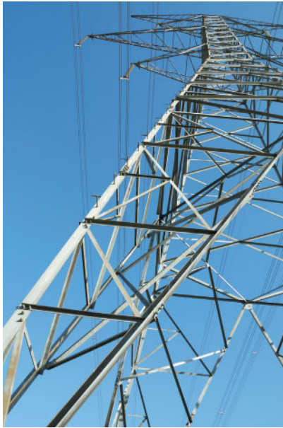
Space trusses are used in the design of many transmission-line towers.
